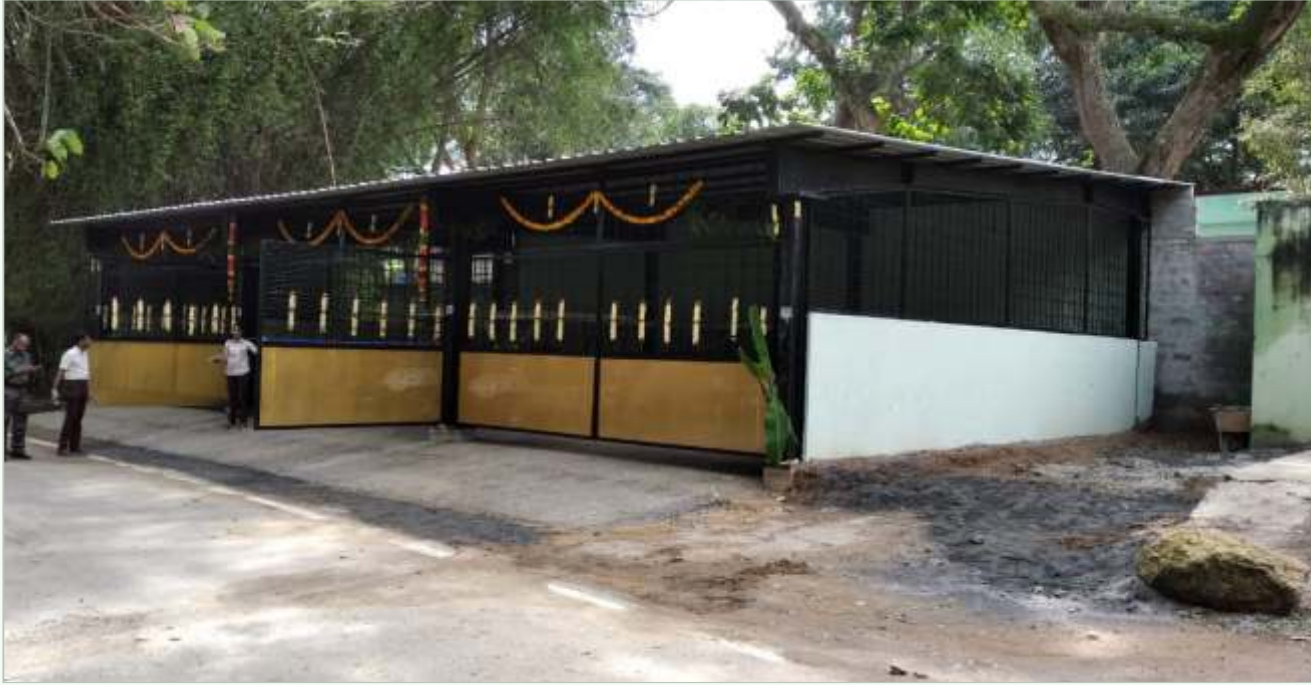
Battery Vehicle Recharge Unit
